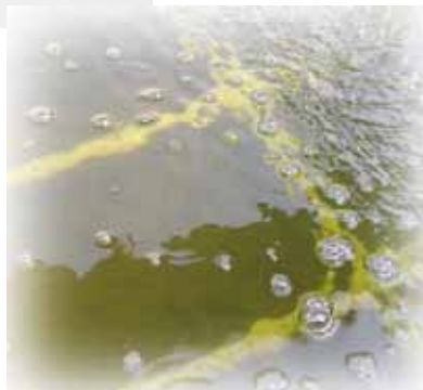
Water entering the slow sand filter via distributed pipe system with maximum aeration
