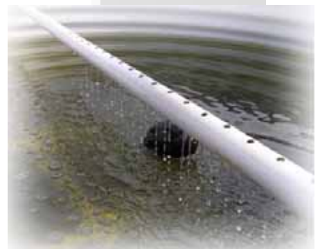
Filtered water entering filtered water tank ready for blending with fresh water stream
